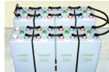
Fig. 5–15: Using row connectors and step connectors
